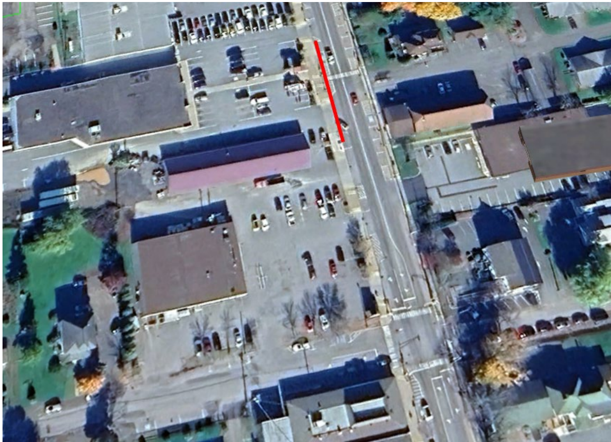
Figure 1: Approximate location (red line) of the unpassable section of 8in gravity sewer line on Commercial St. For reference, the Commercial St / Union St intersection is shown. The section of unpassable line is approximately 45m (147 ft) in length.
